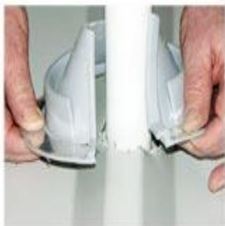
2 Wrap the ZipSeal around the pipe
