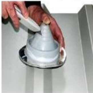
1 Cut to pipe diameter marked on flashing with scissors or trimming knife
