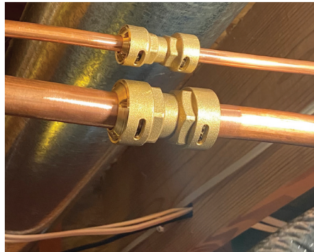
Gino LoPresti, lead HVAC installer with Schar Heating & Cooling, uses ZoomLock PUSH push-to-connect refrigerant fittings on a residential installation for Shawn Stover, Sporlan sales engineer.
