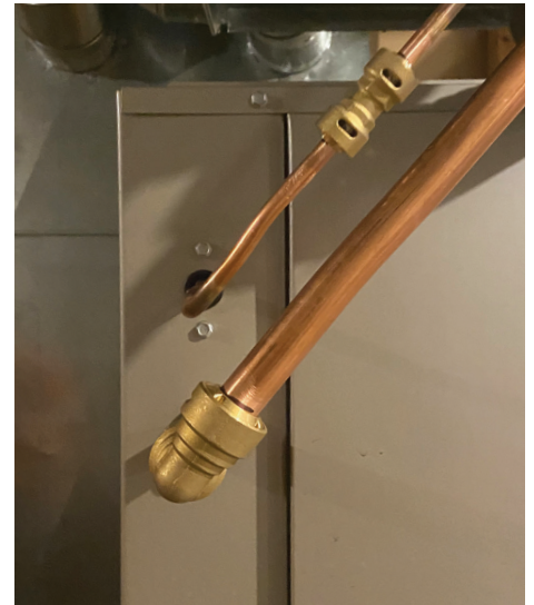
Gino LoPresti, lead HVAC installer with Schar Heating & Cooling, uses ZoomLock PUSH push-to-connect refrigerant fittings on a residential installation for Shawn Stover, Sporlan sales engineer.
