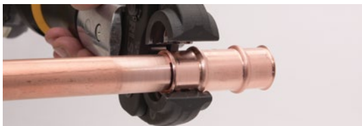
1. Insert the tube in the fitting
